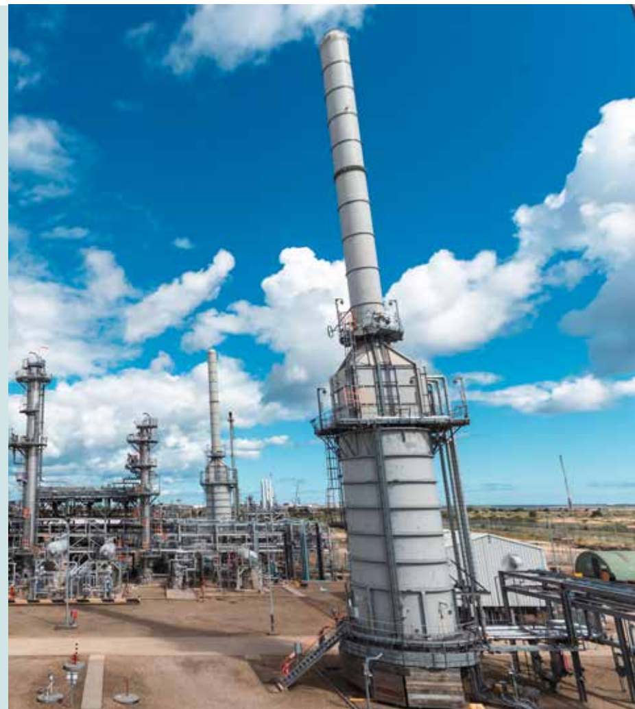
Hot oil heater at the CATS terminal
